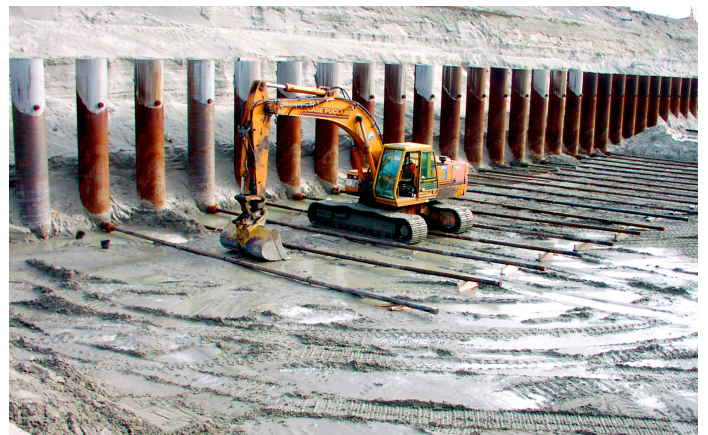
Installation of tie back system
