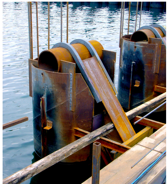
Connection detail of flap anchor
