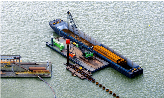
Installation of a tubular combined wall from water
