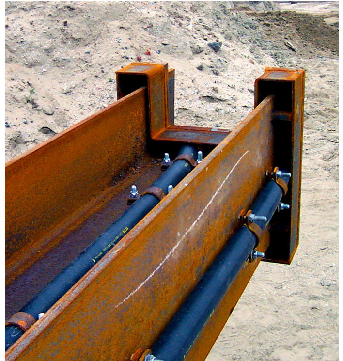
Example of a H beam equipped as MV pile
