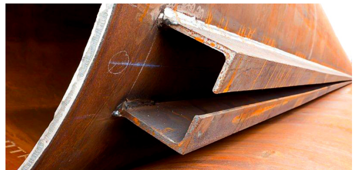
L sections of LT interlock
