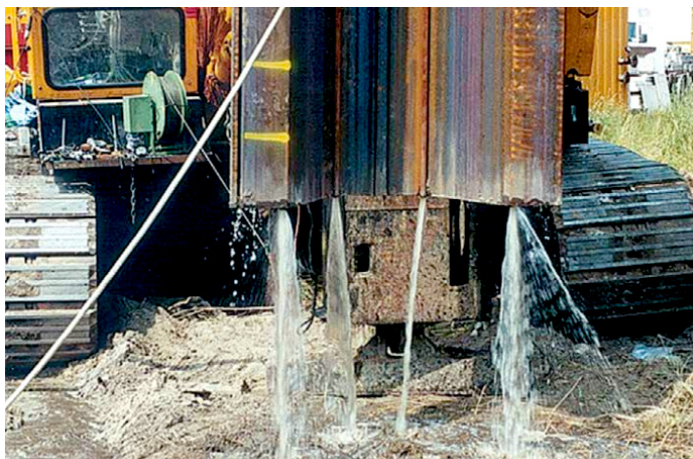
Toe of sheet pile with waterjetting in action.
