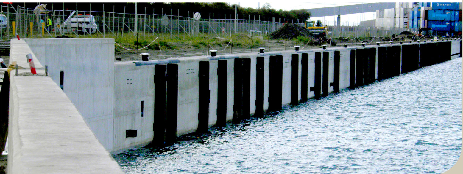
Concrete capping beam in Amazonehaven, the Netherlands
